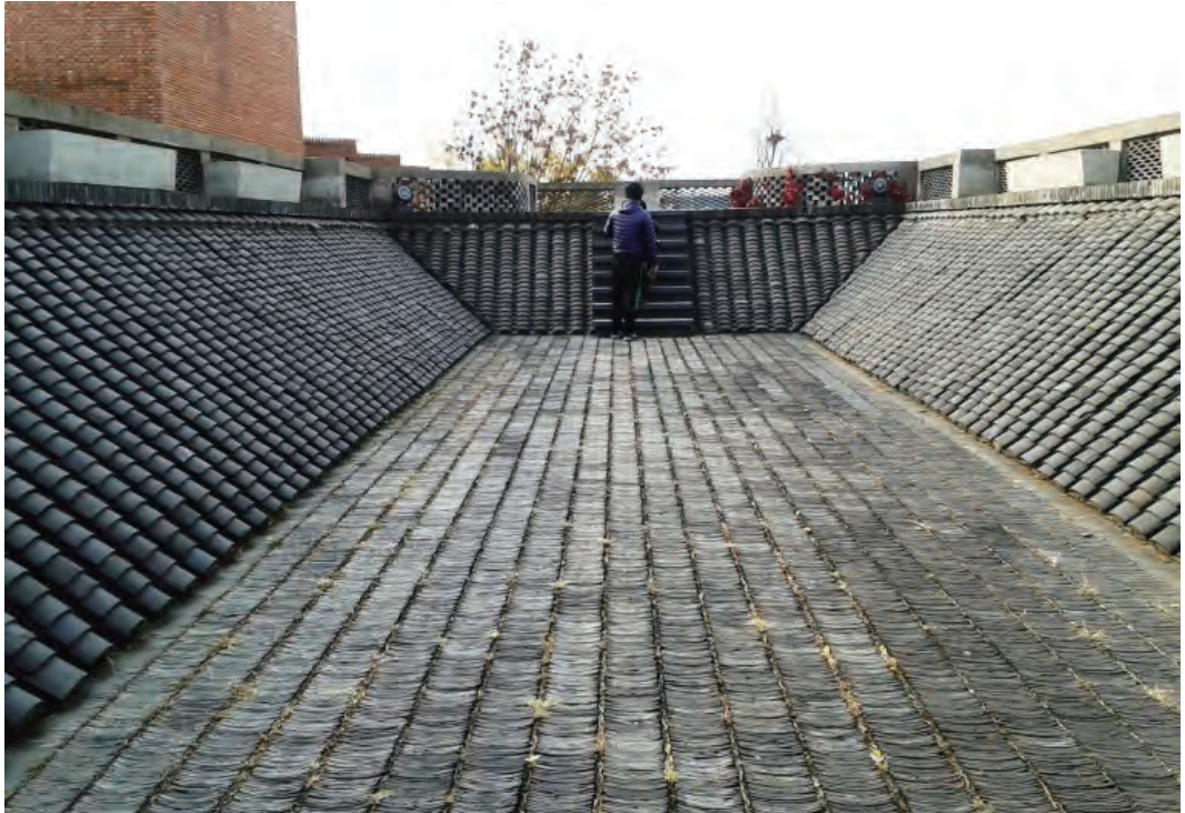
Figure 20. Newly-built V-shaped roof above the lecture hall (Photo: Author)
