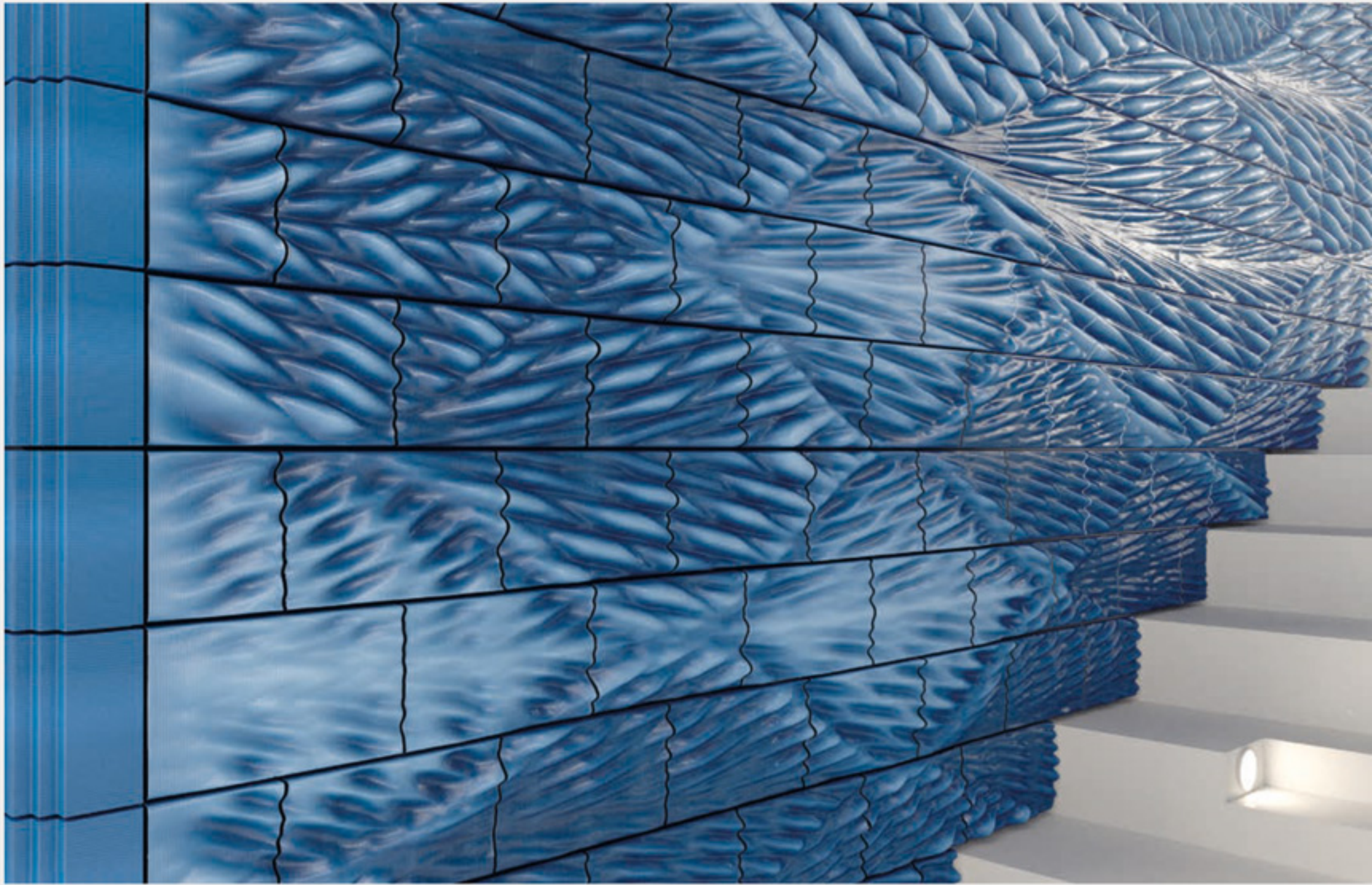
Figure 6: Around 4,000 tiles that will cover the two gates. 3D-printed ceramic is a high-quality cladding material that requires low maintenance and offers high durability.
