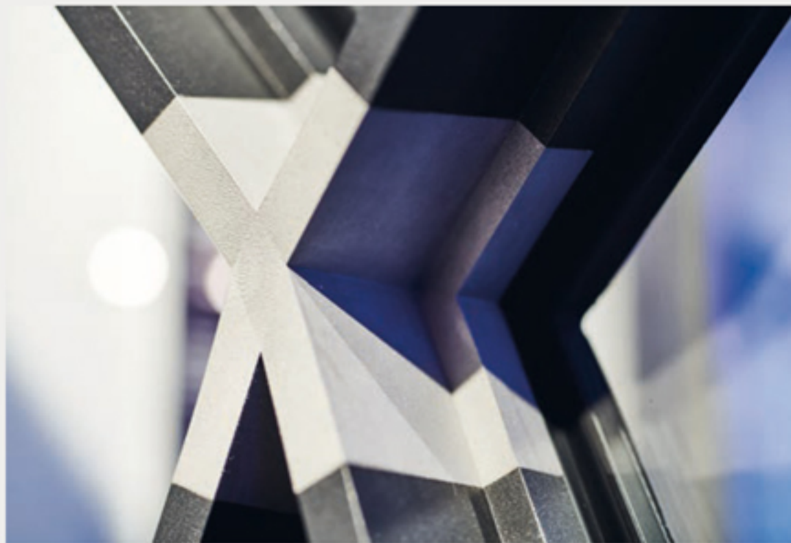
Figure 2: Façade mockup featuring a 3D-printed node
